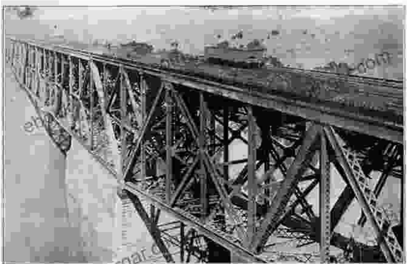
Bridge Shortly After Completion
